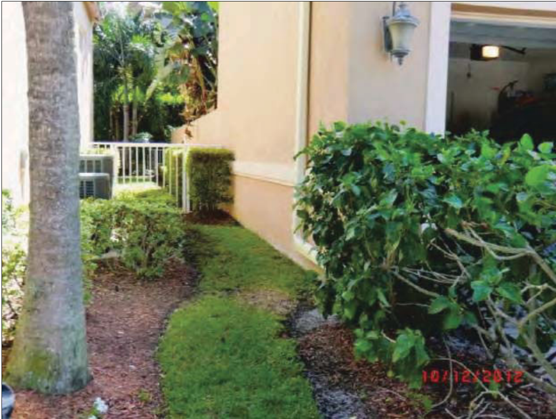
Exterior Finish Condition
